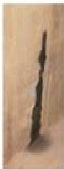
Grease Leakage Outside Containment Wall
