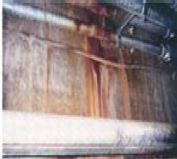
Concrete Wall Water Infiltration
