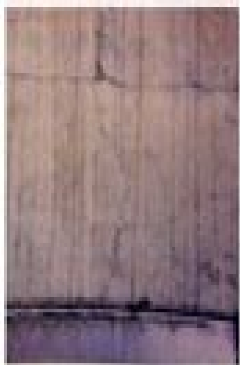
Concrete Cracking Outside Containment Wall
